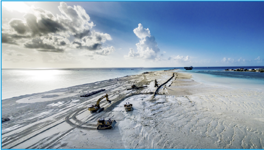
Dredgers raising a Maldivian embankment with Van Oord dredging operations in the background. Courtesy of Van Oord.
